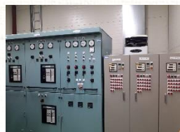
Parallel Panel 2000kW x 3set /380V
