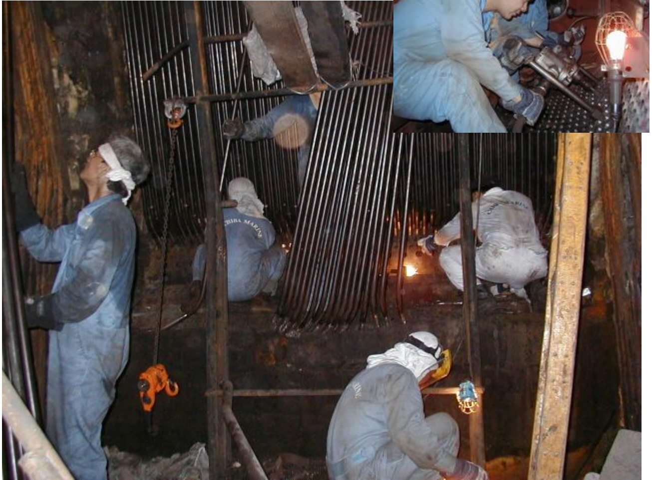
New tubes installation
