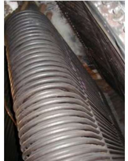
New Superheater in place
