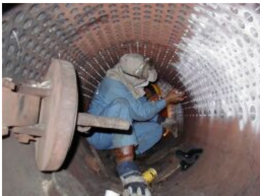
Tube plate dye-checking
