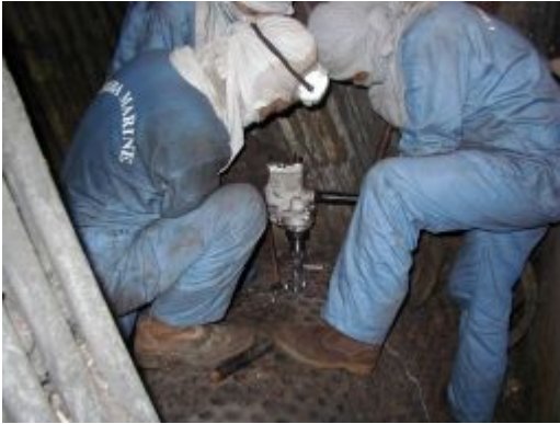
Polishing tube plate
