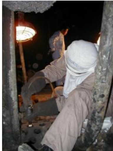
Cropping Damage tubes
