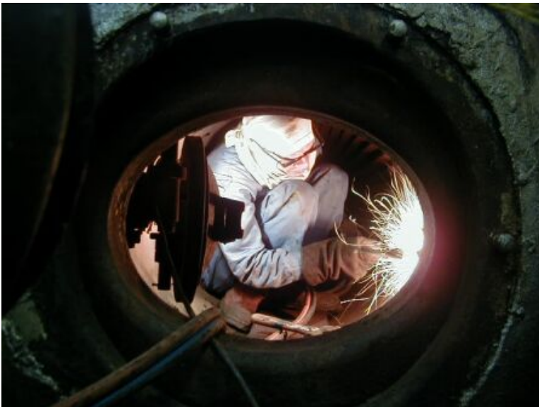
Cutting Damage tubes
