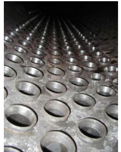
After install tubes
